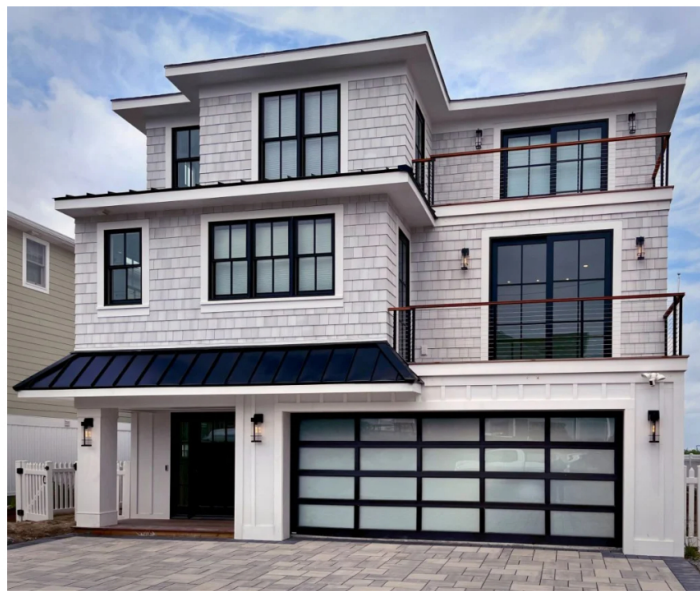
Private Residence in Fenwick Island
